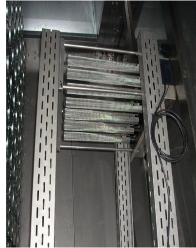
Picture 2 and 3 shows an AerO 3 ACS-I with the downstream equipment Ionisation . Holding Graz: Air Purification 20.000 m 3 /h
