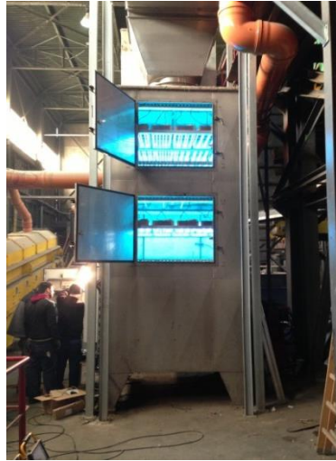
Picture 2 and 3 shows an AerO 3 ACS-I with the downstream equipment Ionisation . Holding Graz: Air Purification 20.000 m 3 /h
