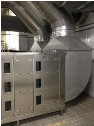
The first Picture shows an AerO 3 ACS-I Berliner Wasserbetriebe Air Purification 2 x 15.000 m 3 /h
