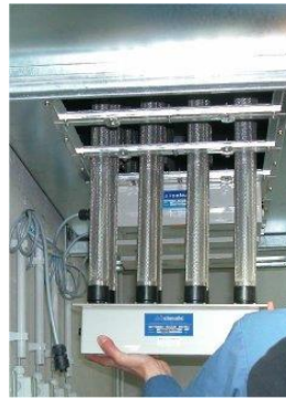
AerOtron - installation in a central ventilation station.
