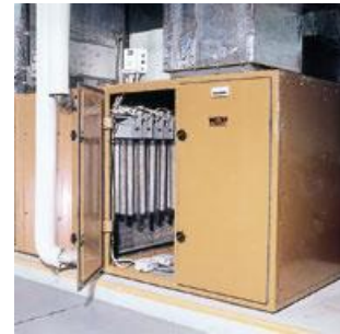
AerOtron - installation in a ventilation duct.
